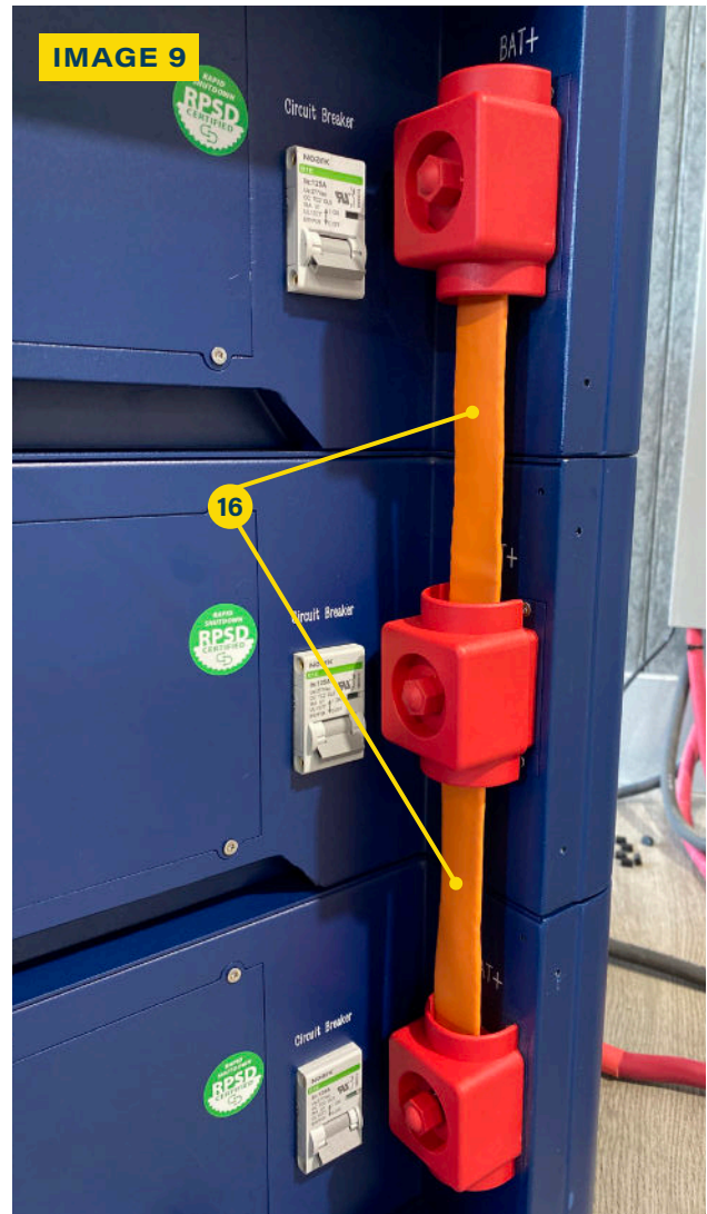
16 PARALLEL BATTERY CABLE
